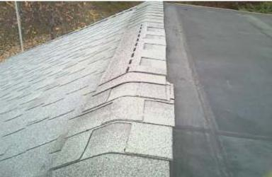
**Missing/cracked shingle** --- Roof has missing or cracked shingles that should be repaired by a qualified roofing contractor. Water penetration could occur at these areas. Have the contractor further evaluate the roofing system for repairs. Location: RIDGE CAP
