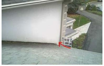
**Elevated moisture ---** There were elevated moisture readings at the below noted location. Elevated readings could indicate an active moisture concern or raise the likelihood of mold, mildew, and/or dry rot. Determine the source of the moisture and correct. Location: RIGHT OF CAR DOOR
